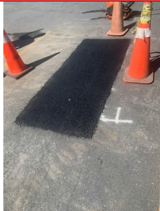
Figure 4: Example of hot-mix asphalt placement
