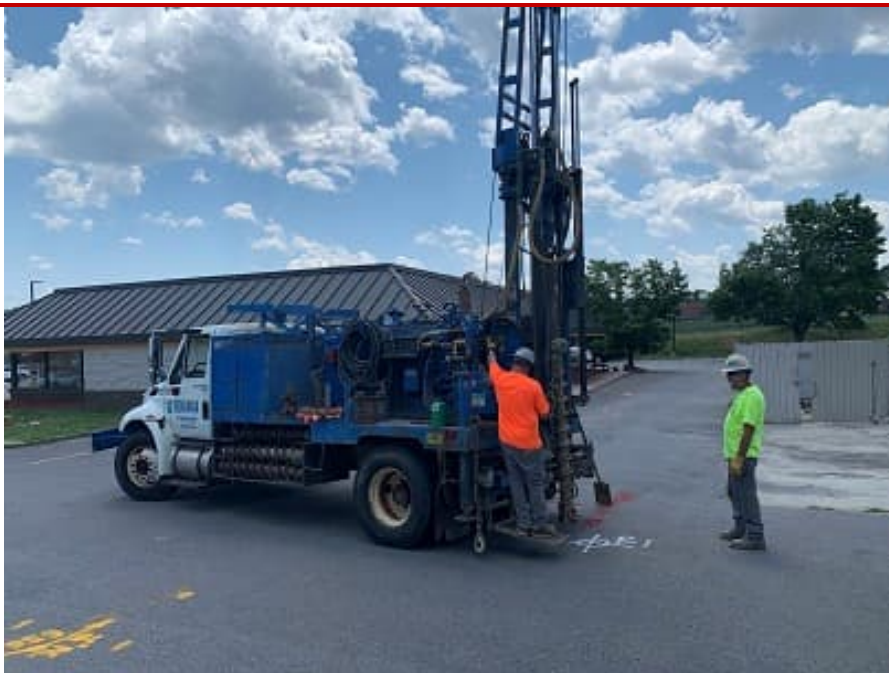
Figure 6: Drill rig setup at P-1
