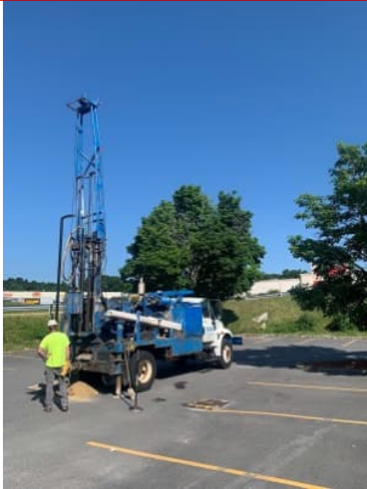
Figure 1: Drill rig setup at B-1
