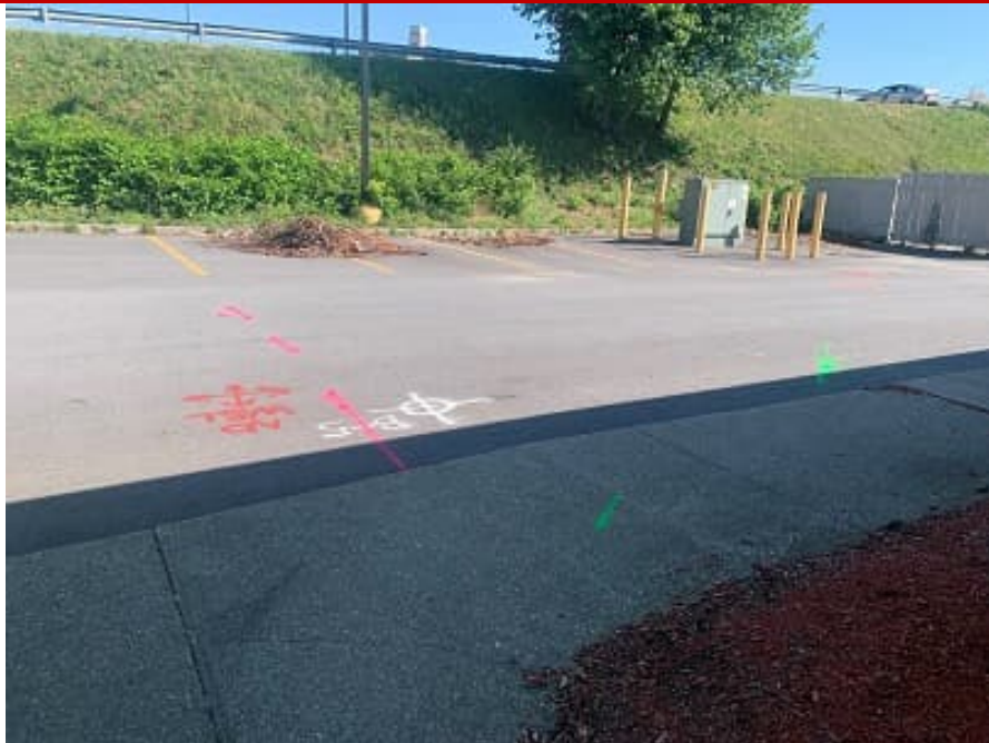
Figure 5: Private utility markout near B-5
